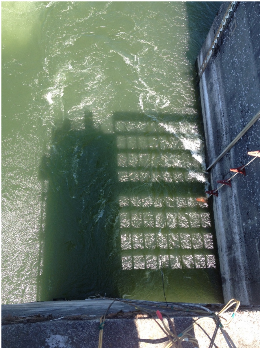
A. 24% valve opening on 7/9/14 (TW = 19 ft) . No visible bubbles from LFS entrances or main flume structure (south wall).
